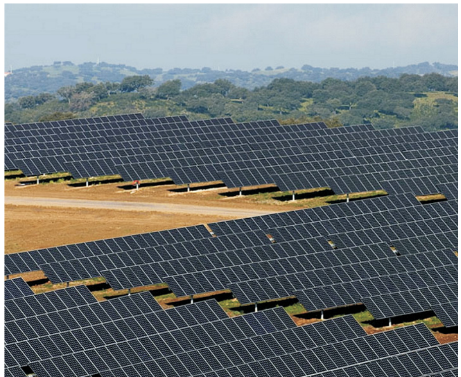
Anlage Application Application Serpa Solar Power Plant (PT)
