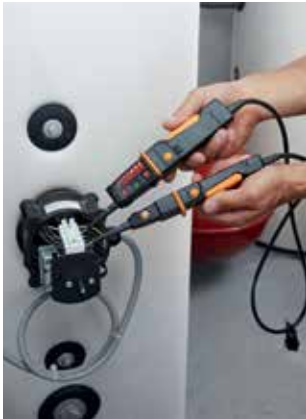
Measuring voltage on a boiler.
