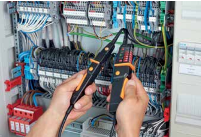
Measuring voltage in a switching cabinet.
