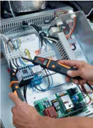
Measuring voltage on a compressor.
