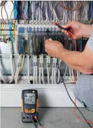
Testing voltage in a switching cabinet.
